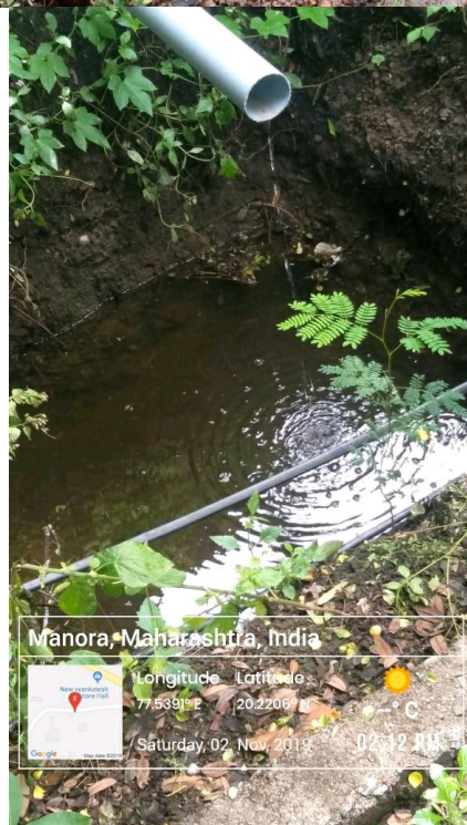
Photo: Showing down water pipe system for Recharging of rain water behind Library
